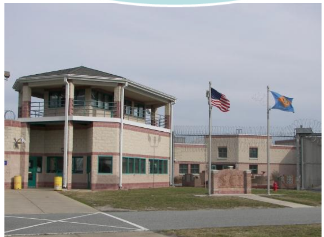
Sussex Correctional Institution Opened: 1931 Operating Capacity: 1,149
